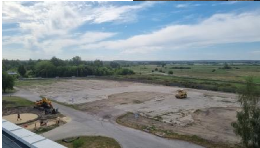
Land cleared for solar park Kozenice, Poland
